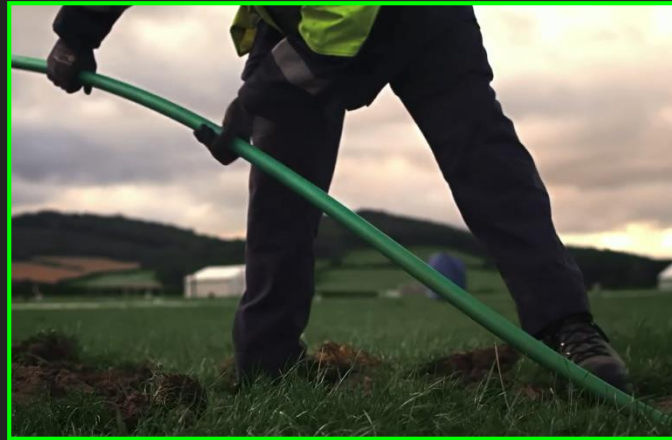
Home passed feeder cable can lay along existing ducts, to minimize the excavation
