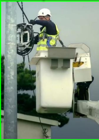
Home passed feeder laid along distribution lines and terminated at fixed cabinets on the utility pole
