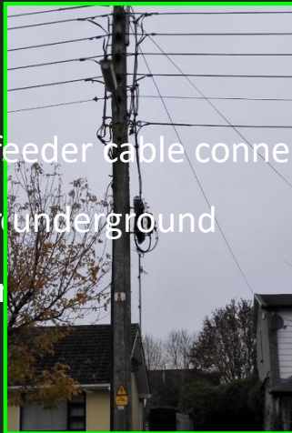
Home passed feeder laid along distribution lines and terminated at fixed cabinets on the utility pole
