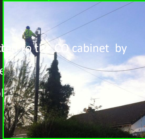
Home passed feeder laid along distribution lines and terminated at fixed cabinets on the utility pole
