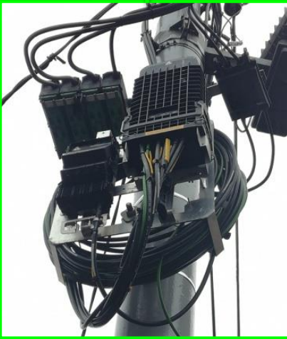
Home passed feeder laid along distribution lines and terminated at fixed cabinets on the utility pole
